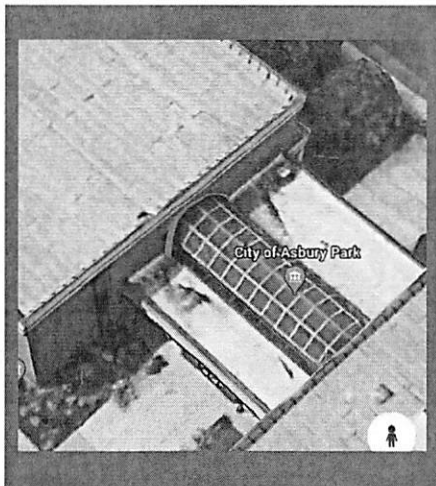
South wall area of concern
