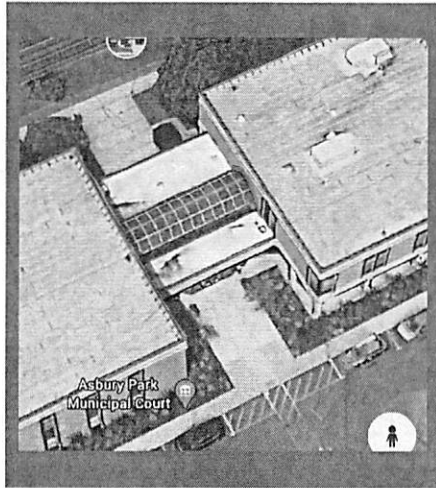
North wall area of concern
