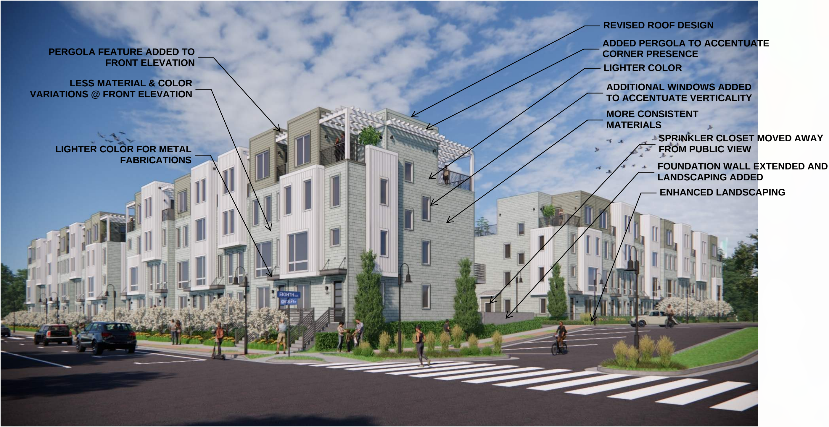
BUILDING #3 & #4 - INTERSECTION OF KINGSLEY STREET AND EIGHTH AVENUE
