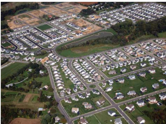
Aerial Photo (under construction)
