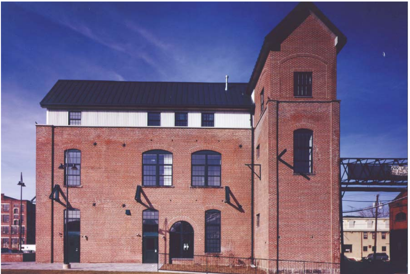
View from Roebling Complex entry
