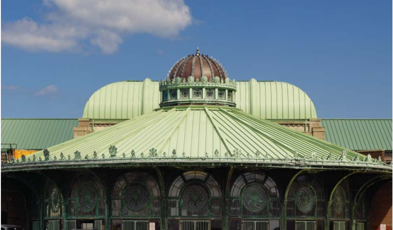
Carousel House Rooftop
