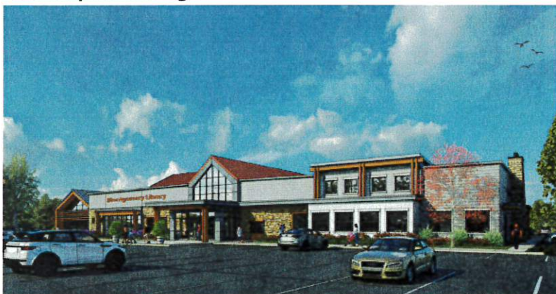
Library Main Entrance
