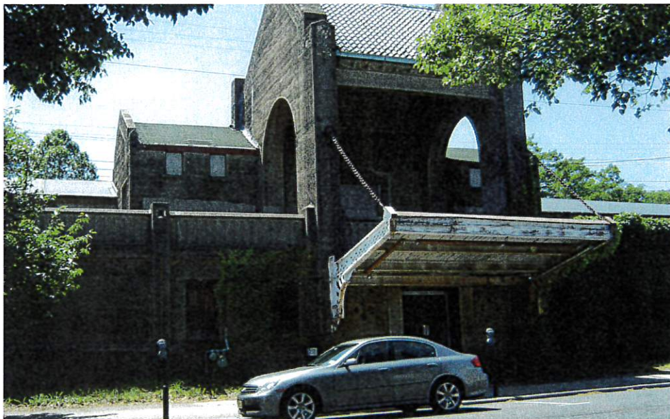
Existing Bloomfield Train Station
