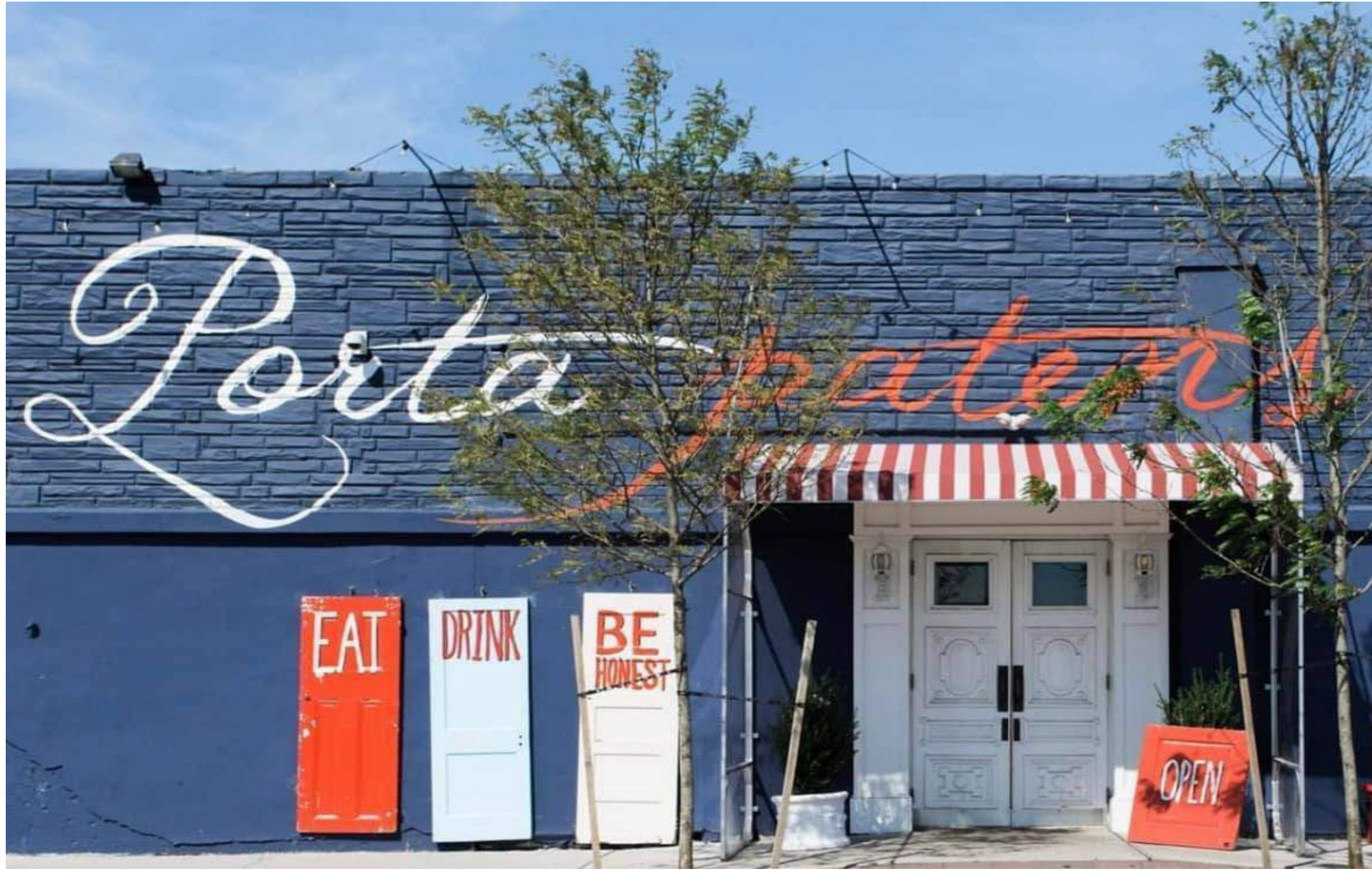
EXISTING BUILDING FACADE
