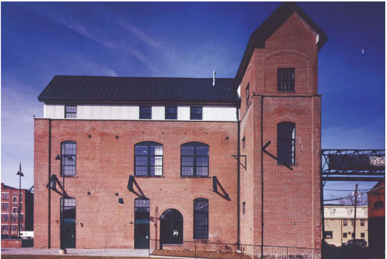
View from Roebling Complex entry
