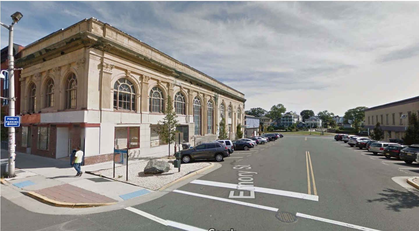
VIEW ON EMORY ST. LOOKING SOUTH
