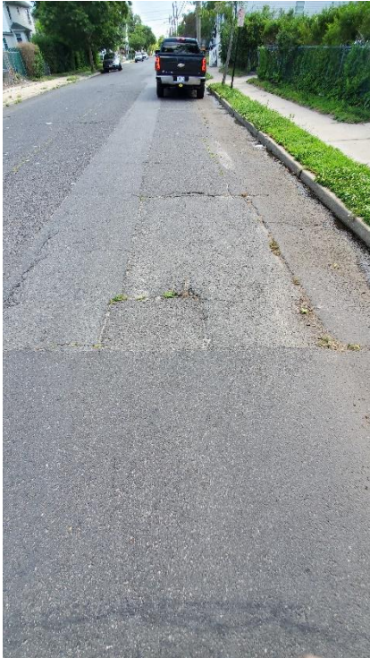
Roadway Patches and Trenching
