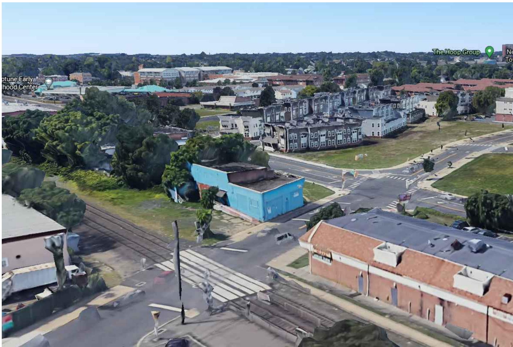
8 EAST CORNER AERIAL VIEW SCALE: NTS
