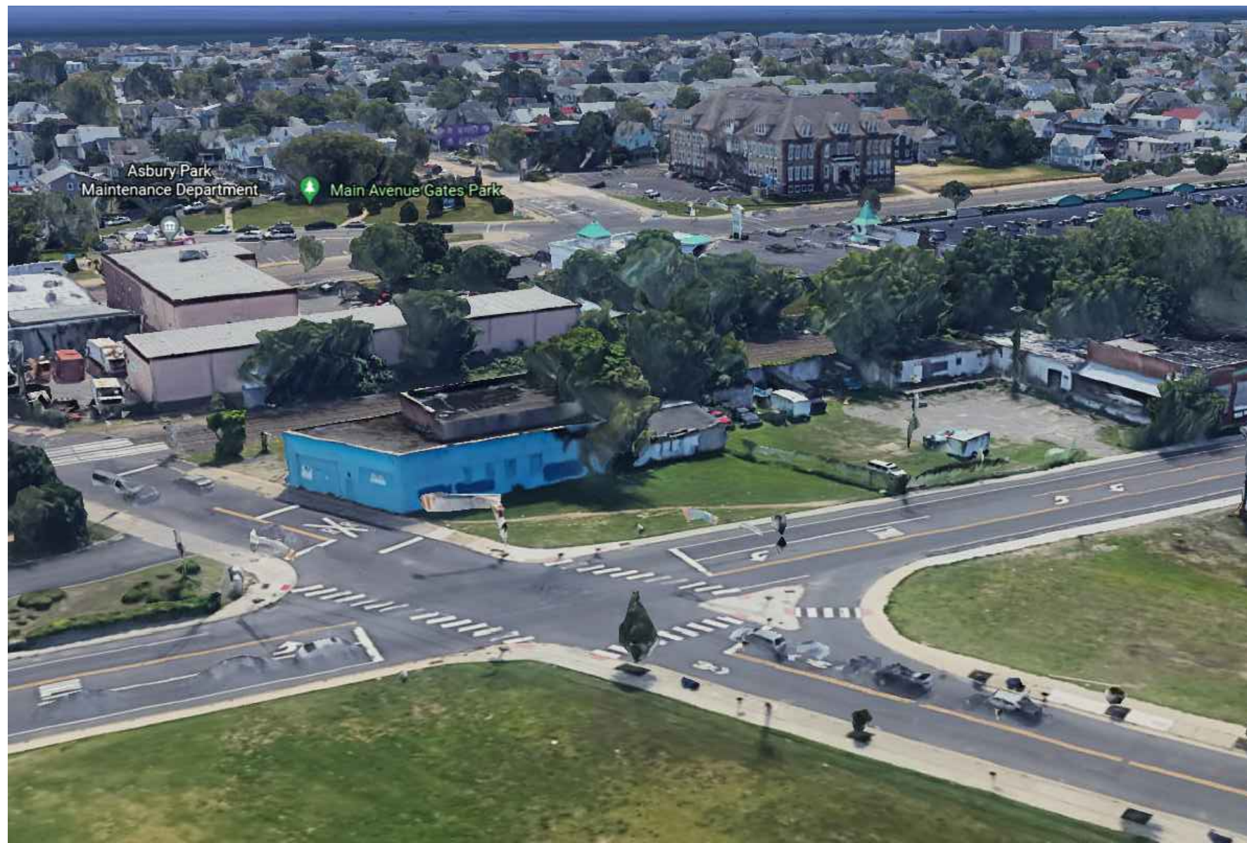
9 NORTH CORNER AERIAL VIEW SCALE: NTS
