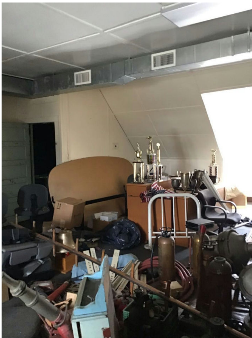
12 12-Pre-Mitigation - Document Date Taken: 7/16/2021 Room (Zone 1) 9
