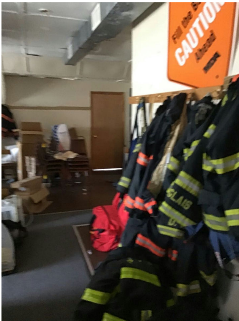
5 5-Pre-Mitigation - Document Date Taken: 7/16/2021 Room (Zone 1) 2
