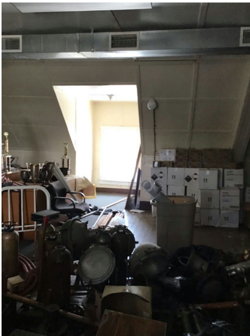
13 13-Pre-Mitigation - Document Date Taken: 7/16/2021 Room (Zone 1) 10
