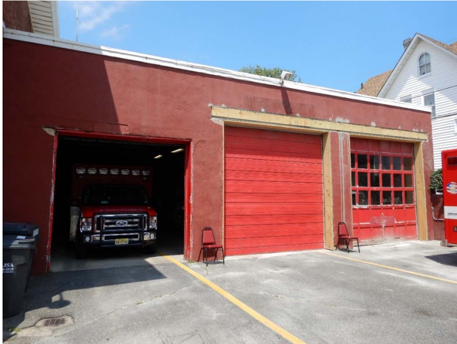
Bay door #1 left of the two repaired bay door lintel positions.
