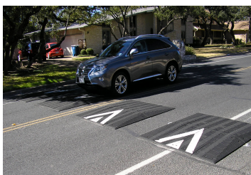
Gaps Between Great for Fire Truck Passage
