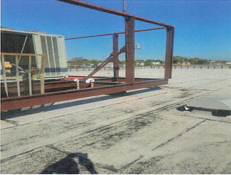
overview roof area
