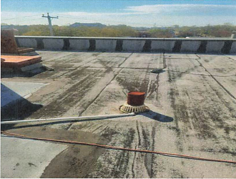
overview roof area
