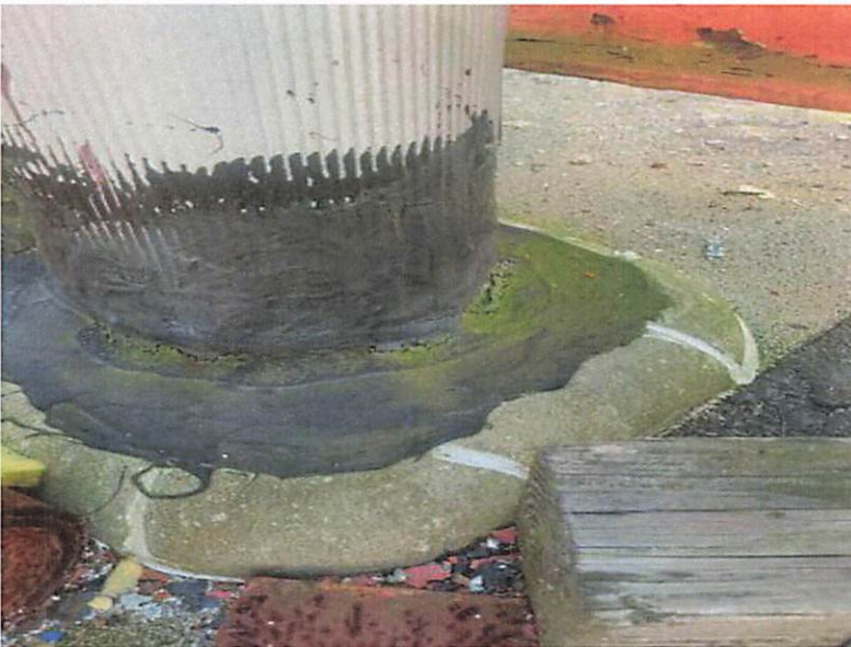
open sealant at pitch pocket
