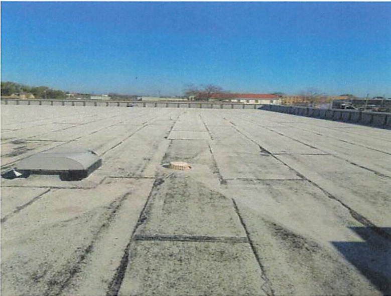
overview roof area
