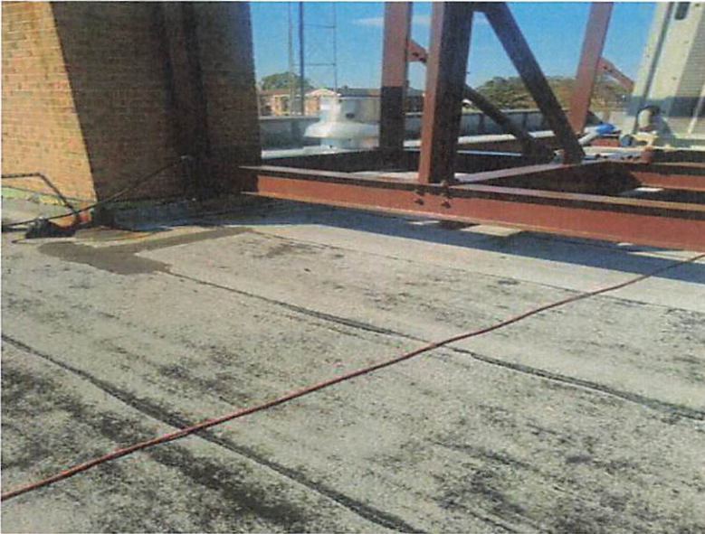
overview roof area
