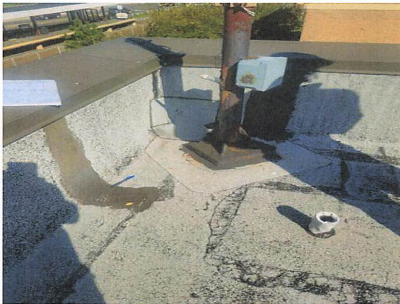
inside northwest corner
