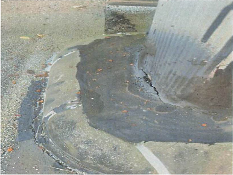
open sealant at pitch pocket
